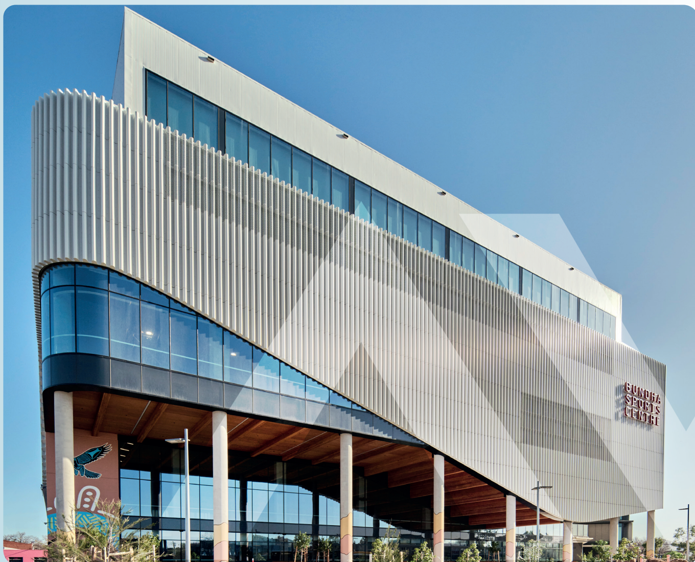
Bhunda Sports Centre in Victoria is Australia's first publicly accessible vertical sports centre
