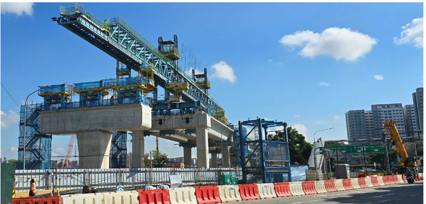
Inland Rail project, Victoria, tranche 1 works being delivered by McConnell Dowell.
