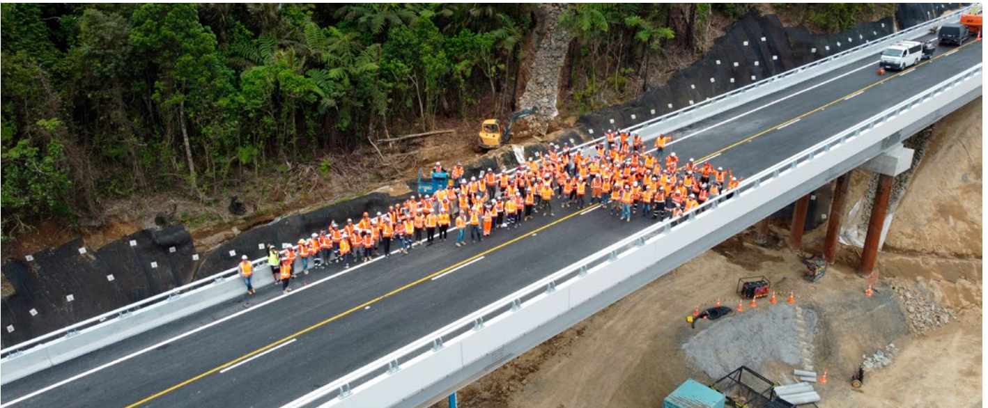
State Highway 25A Taparahi Slip Remediation, New Zealand. Awarded "Bridge Project Team of the year" at the New Civil Engineering Awards, London.
