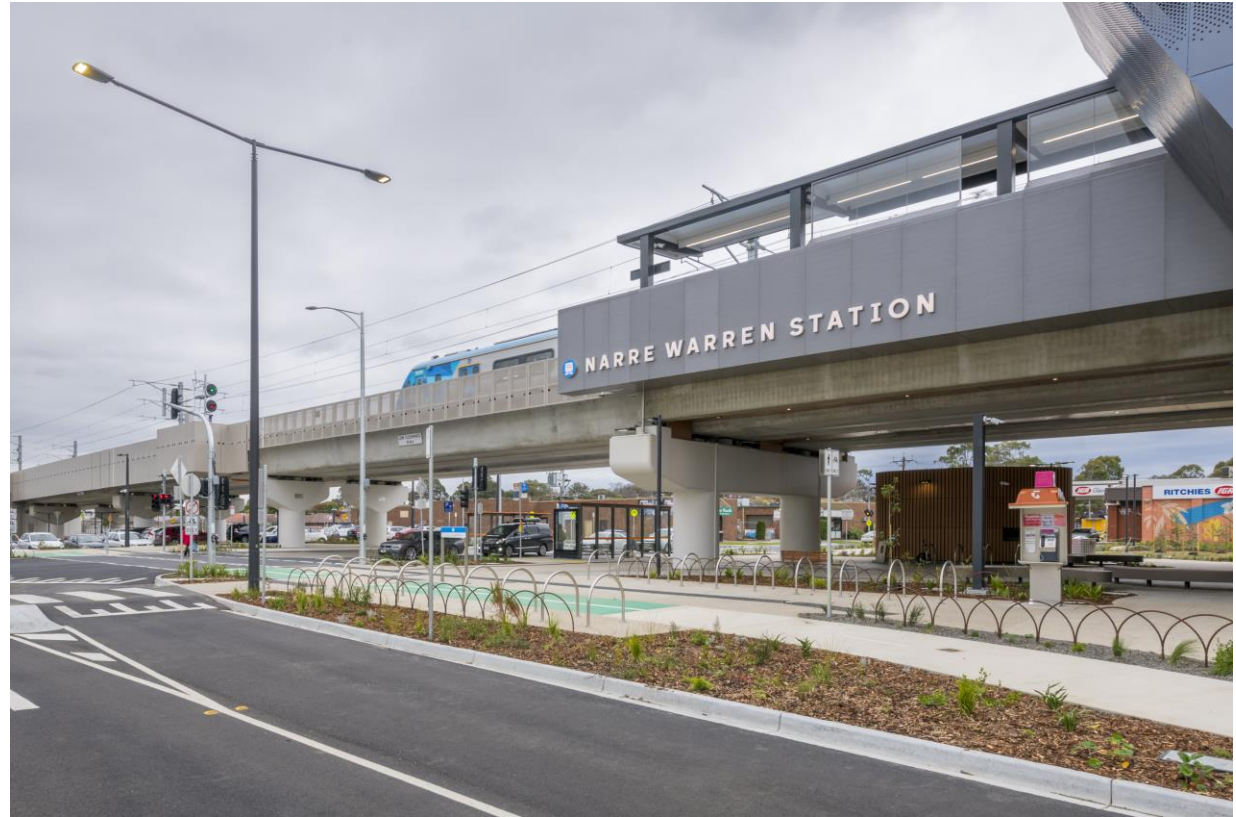
Narre Warren Level Crossing Removal and Station Upgrade, Victoria Another successful collaboration between McConnell Dowell and Built Environs
