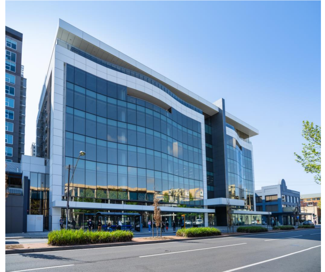
150 Grenfell Street, Adelaide Two ageing office buildings reimagined into an exemplar of sustainability and adaptive re-use
