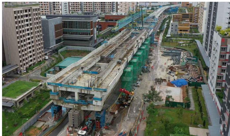
Jurong Regional Line (J108), Singapore Unforeseen brownfield complexity and disruption
