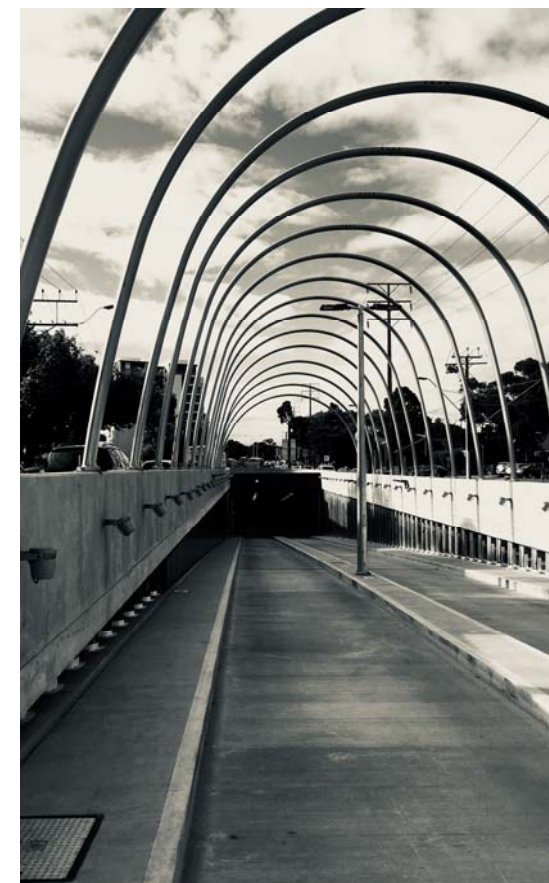
McConnell Dowell's O-Bahn City Access project
