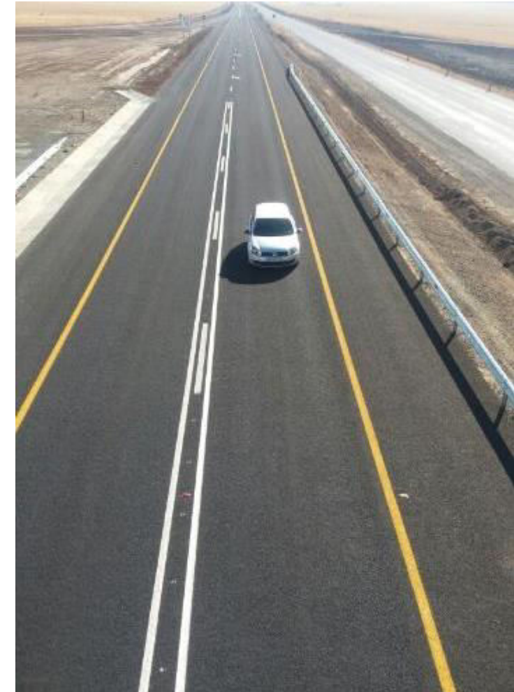
Aveng Grinaker-LTA Ventersburg Roads Project
