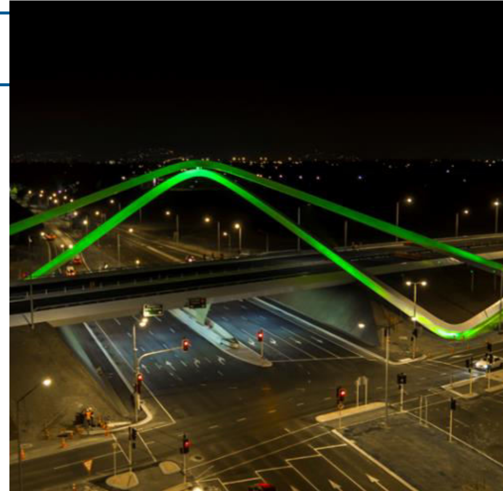
McConnell Dowell, Russley Road, New Zealand
