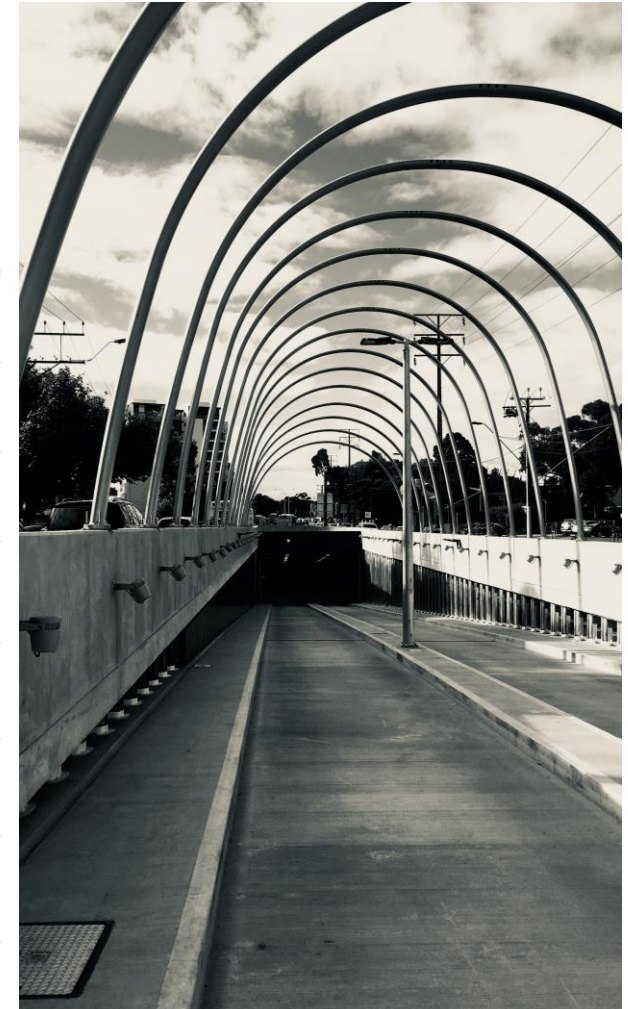
McConnell Dowell's O-Bahn City Access project
