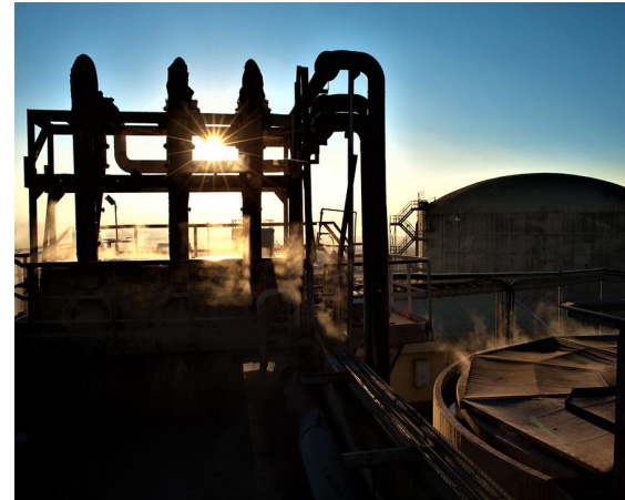
Aveng Water eMalahleni Reclamation Plant
