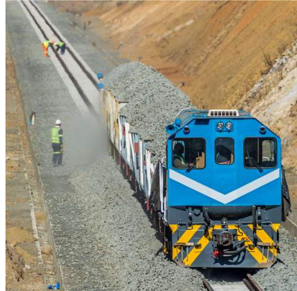
Majuba Rail Project, Aveng Grinaker-LTA Civil Engineering, Ermelo
