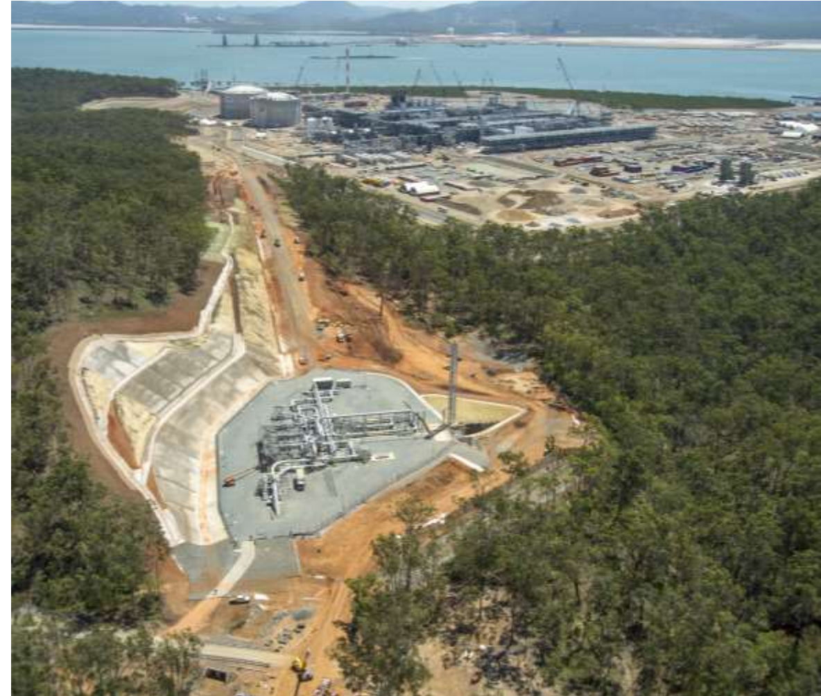
Queensland Curtis Liquefied Natural Gas Pipeline Project , Australia
