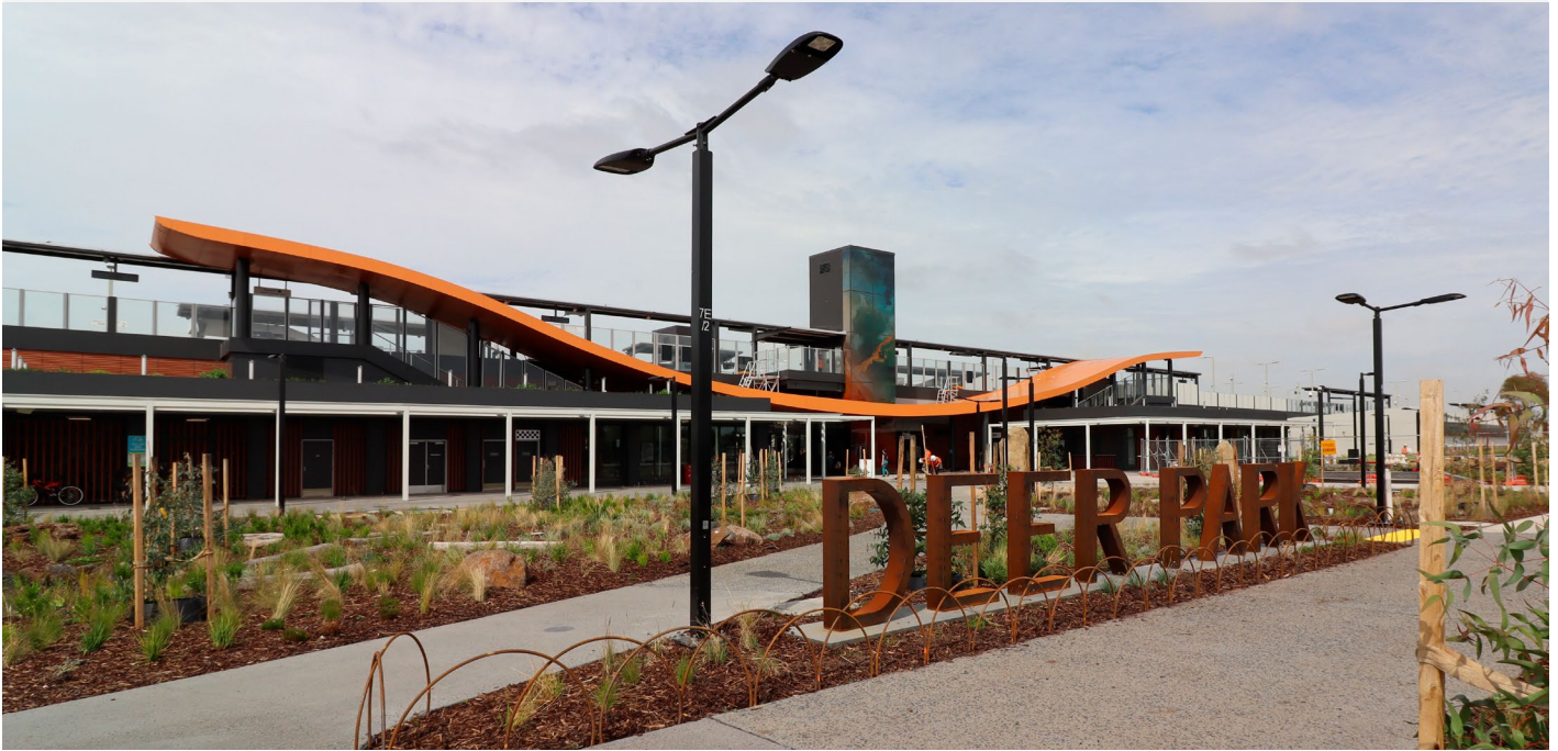
Solar bus shelters at the Deer Park Station in Melbourne generate renewable energy.
