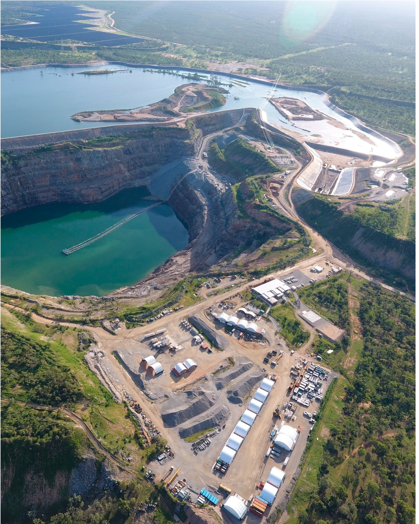
Kidston pumped storage hydro project in Queensland, Australia, converted a disused gold mine into a pumped storage hydroelectric power generation facility.
