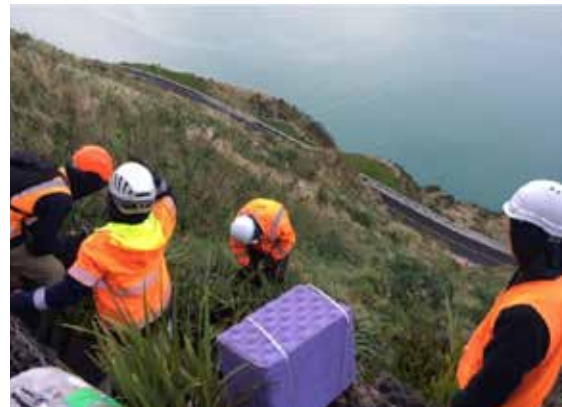
Subcontractors carrying out indigenous planting on the Sumner Road project
