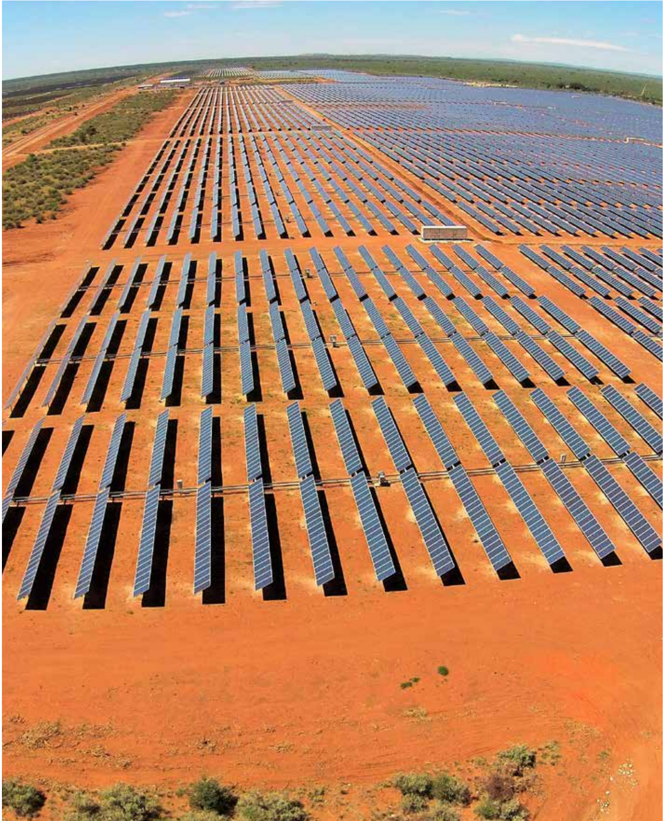
Sishen Solar Farm, Northern Cape
