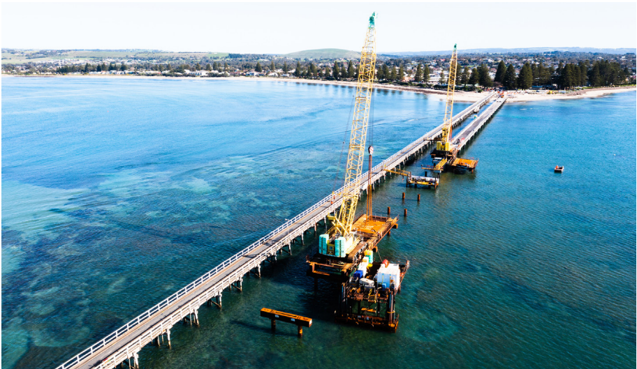
Granite Island Causeway Renewal
