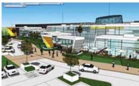
The Mall of the South shopping centre to be constructed in Meyersdal, Johannesburg.
